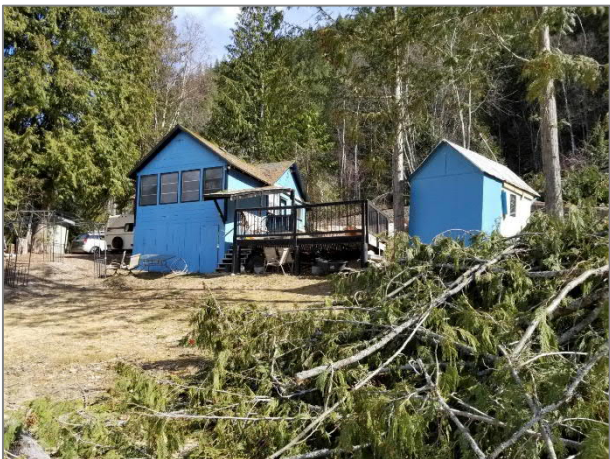
Photo 7. View of one-bedroom cabin, deck and pumphouse.
